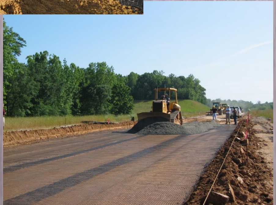
Base Reinforcement (CBR >4)
