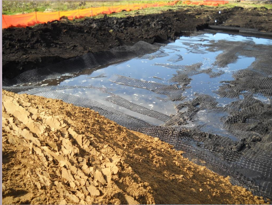
Subgrade stabilization (CBR <4)
