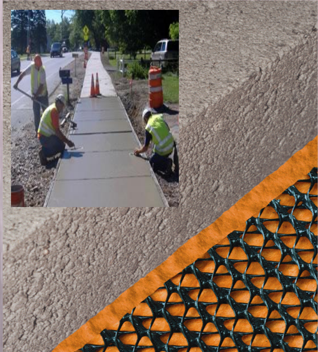
Grave replacement layer for concrete slabs
